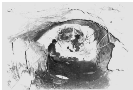
Fig. 1. Underground opening exhibiting side collapse in the form of successive spalling forming a stable breakout shape.
